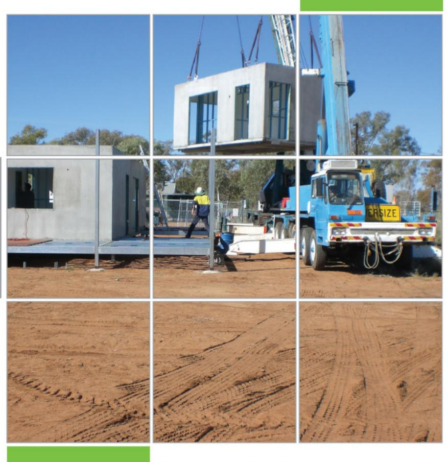
The Green Precast System delivers construction times up to 80% faster than traditional superstructure systems and is ideal for large and repetitious projects where onsite manufacturing delivers optimum benefits.
