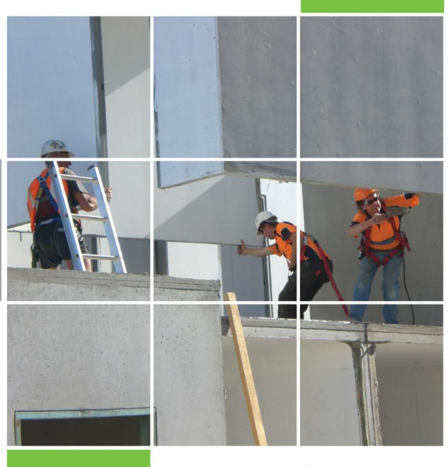
The self supporting system provides a safer work environment than traditional tilt slab construction methods. Requiring no propping, brackets or expensive scaffolding.
