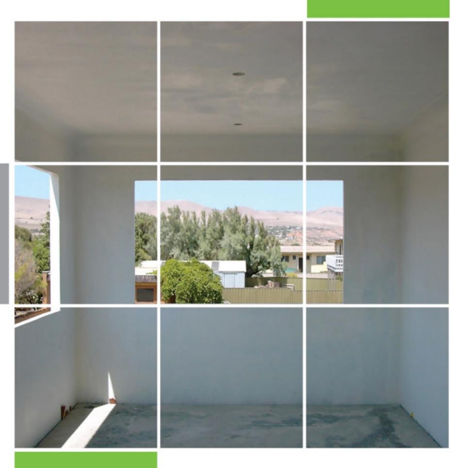
With a Class 1 finish, the off-form quality of wall and ceiling means that plasterwork can be in most instances eliminated.
