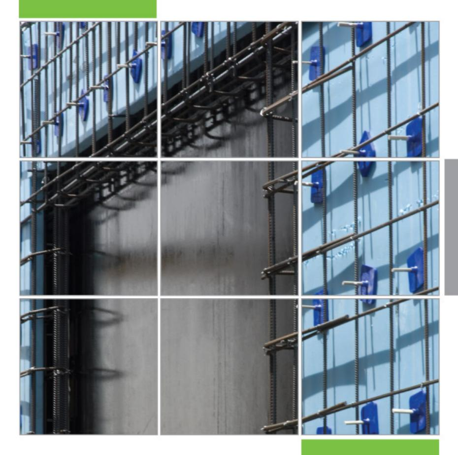
The thermal and acoustic qualities of the modules are tremendous, with insulation being embedded within each concrete sandwich. High tech external finishes can further enhance efficiencies.
